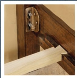
Rail and Slat Dovetail Construction
