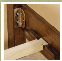
Rail and Slat Dovetail Construction
