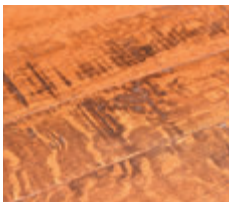
Barn Floor (BF)
